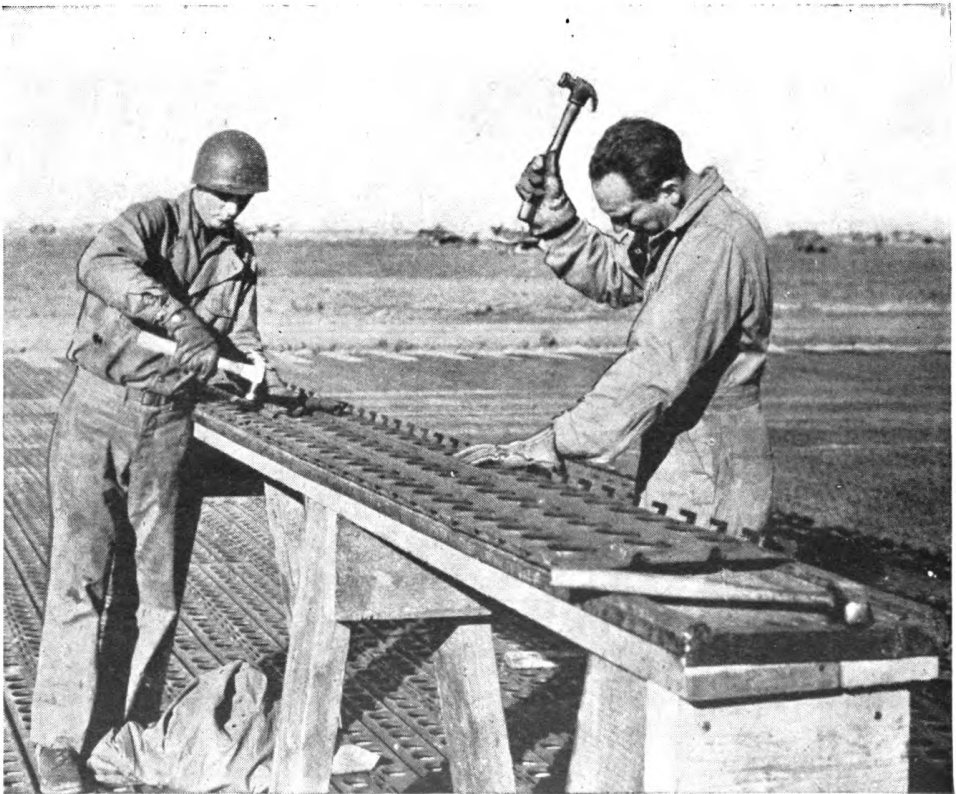
Figure 88. Damaged panels being repaired by hand methods.
